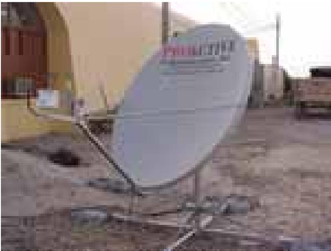
**V SAT (Very Small Aperture Terminal)** are small fixed satellite antennas that provide highly reliable communication means for data, voice and fax between almost any number of geographically dispersed sites.
