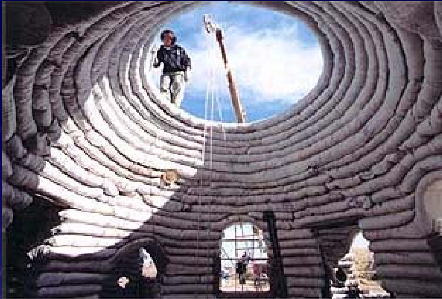
Cal Earth sandbag and barbed-wire “superadobe” shelters
