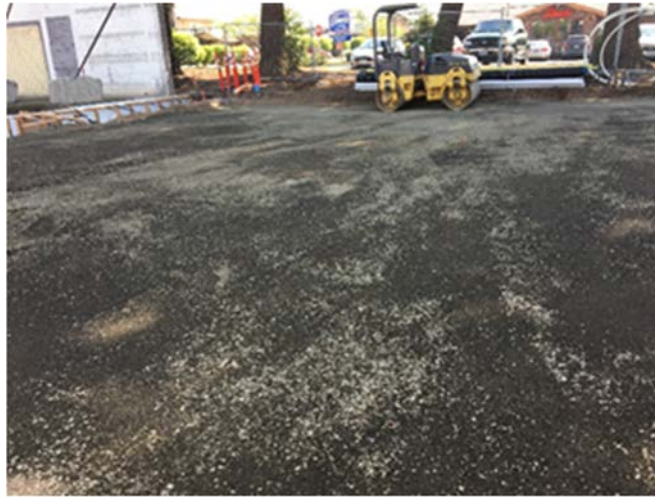
Figure 30. Compacted gravel surfaces prevent the erosion or movement of the underlying subgrade.
