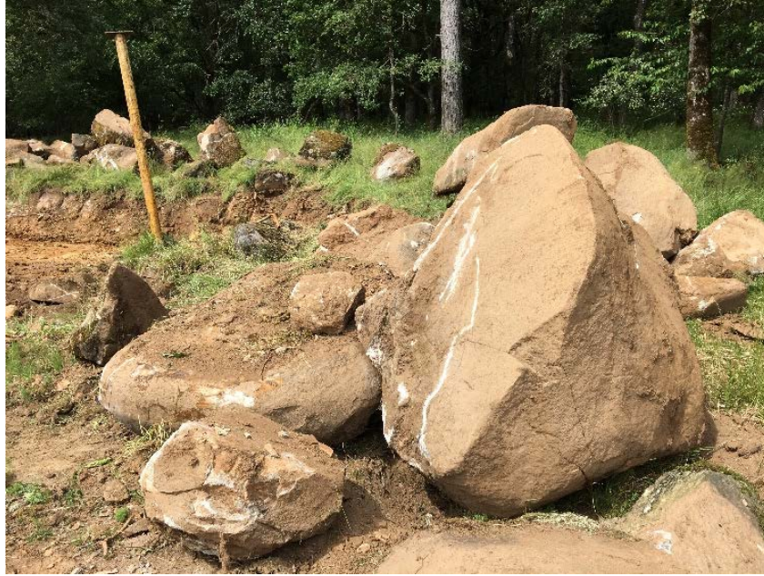
Figure 3. Unknown subsurface conditions, like large boulders, can cause serious delays in construction!
