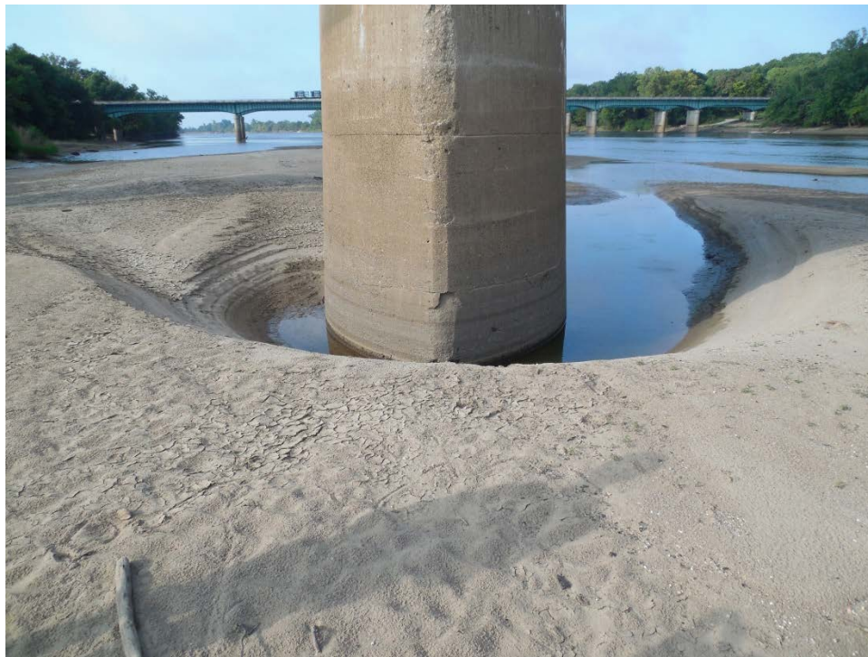
Figure 28. Scour around bridge pier (courtesy of USGS ).
