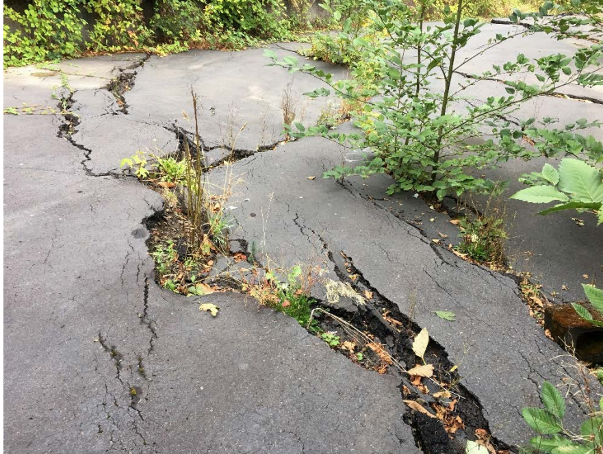
Figure 13. Transverse crack extending through flexible pavement surface.
