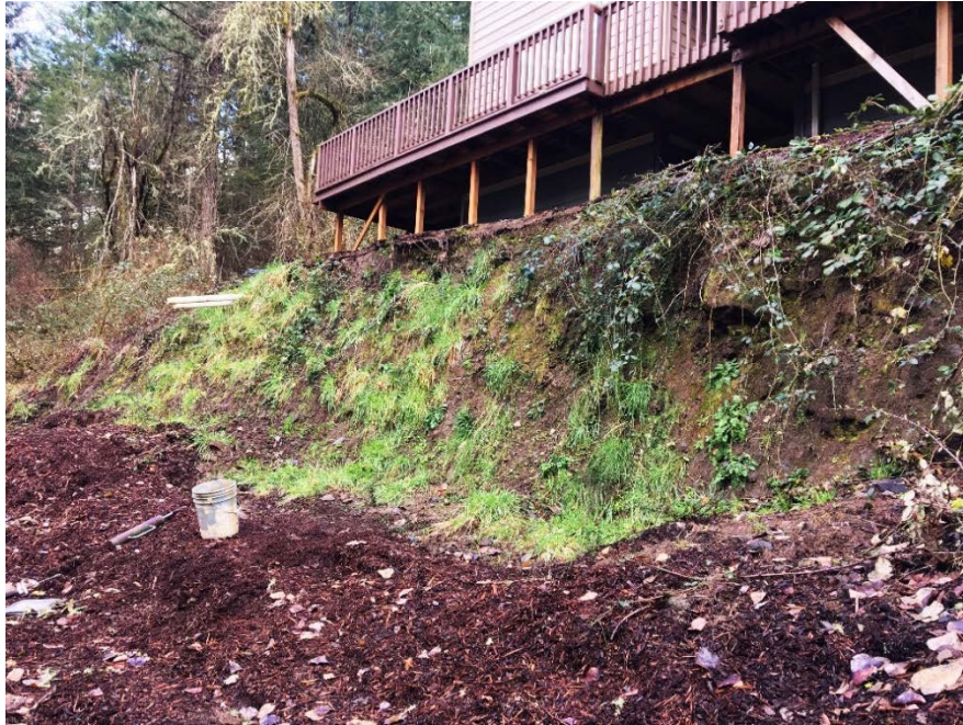
Figure 12. Deep scarps forming behind residential construction.
