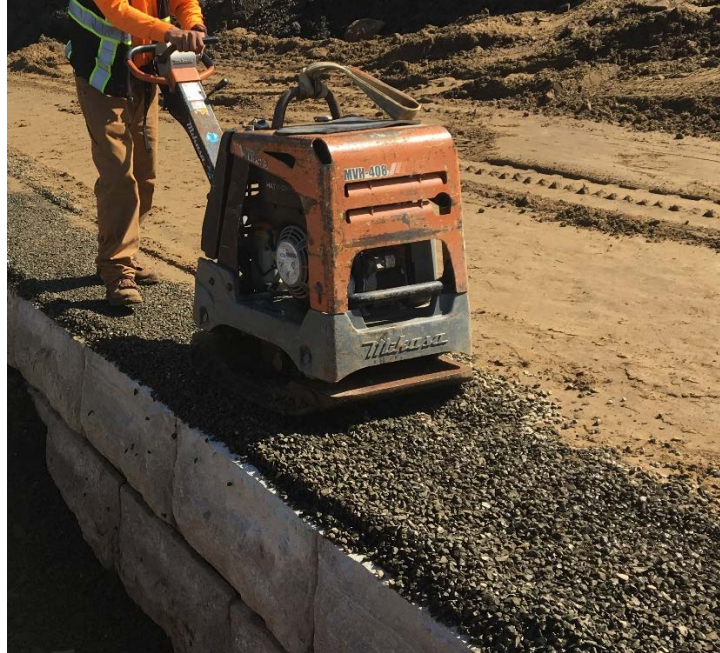
Figure 36. Vibratory plate compactor used to compact gravel fill behind a retaining wall.
