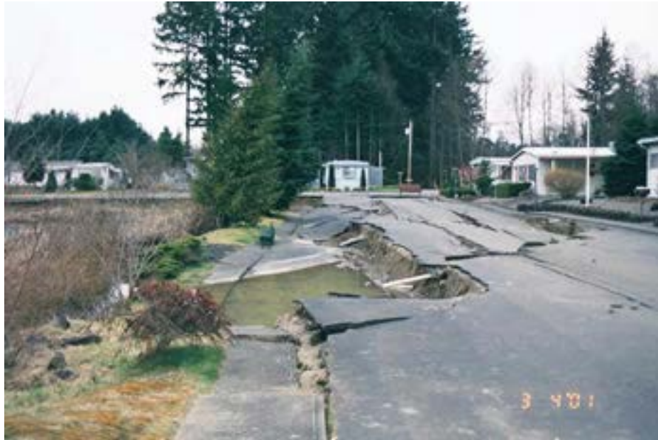
Figure 22. Liquefaction induced lateral spreading (courtesy of Geomatrix )
