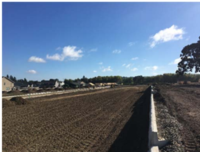
Figure 31. Roughened surface after soil compaction.
