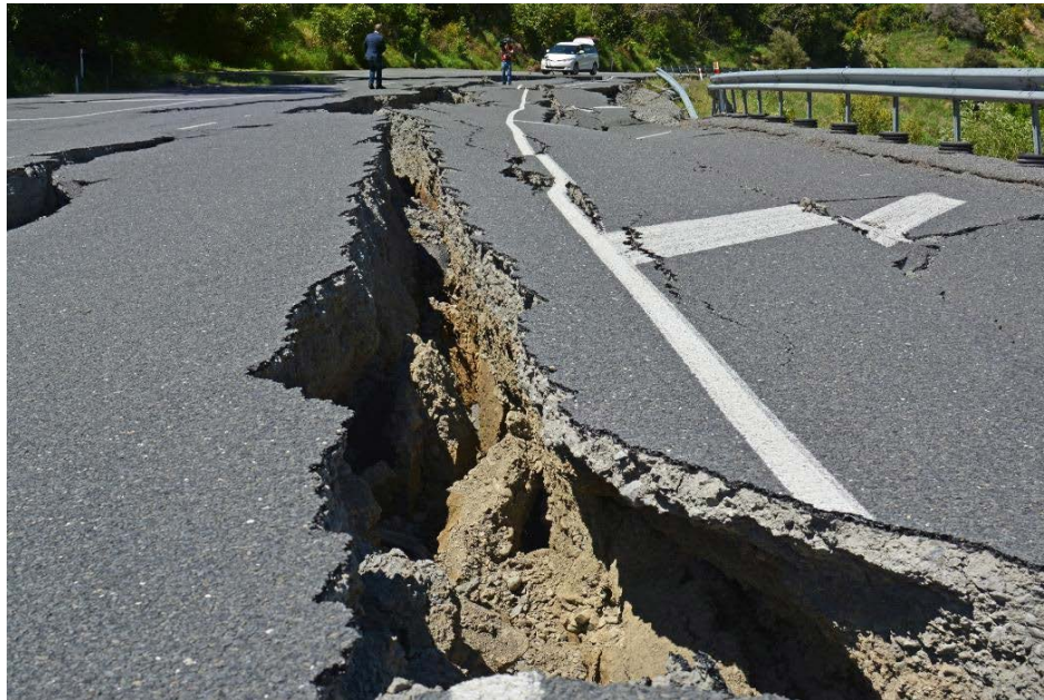
Figure 24. Fault rupture extending to the ground surface (courtesy of newsatlas.com )
