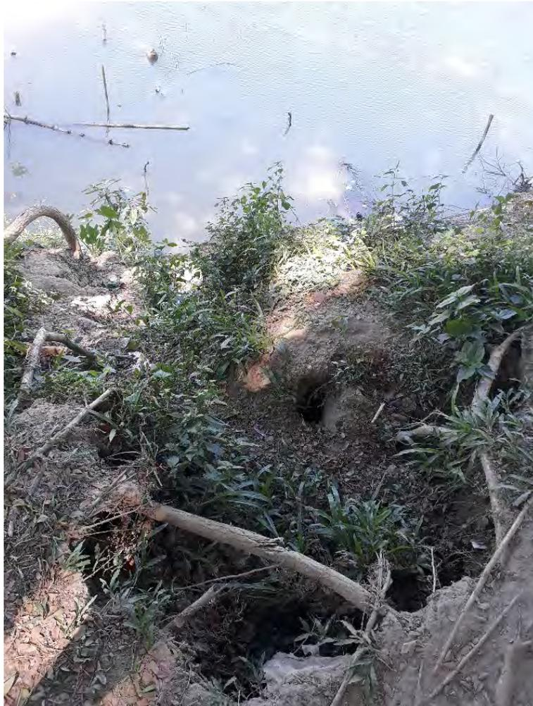
*Photo 3 Scouring from surface water runoff on top of the riverbank*
