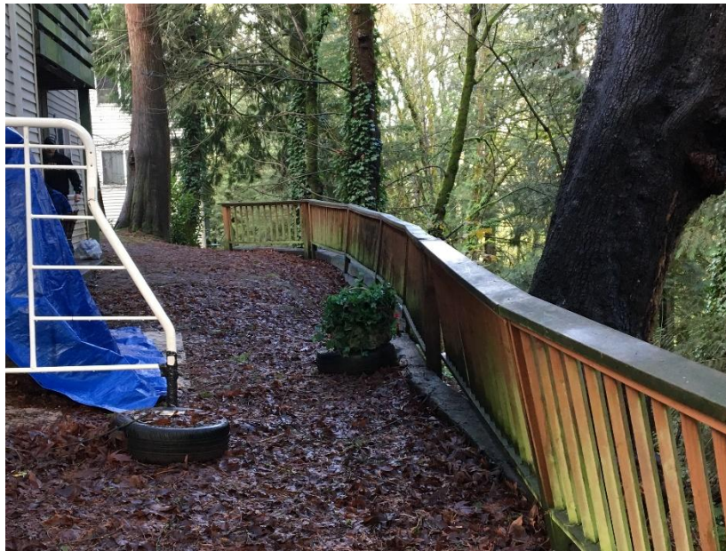
Figure 16. Slope failure resulting in damage to the border rail.
