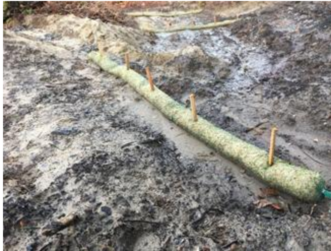
Figure 32. Wattles placed perpendicular to the slope contours. Note the buildup of sand behind the wattle.
