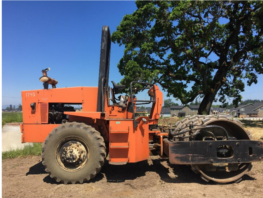
Figure 35. Sheepfoot roller used to compact sandy-silt soil.
