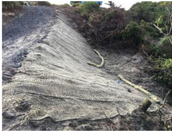
Figure 33. Jute mesh used to protect the slope from rainfall and surface runoff.
