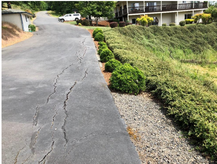
Figure 11. Tension cracks forming parallel to the crest of a slope indicating failure.
