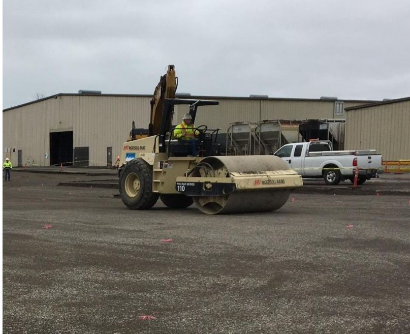
Figure 34. Smooth drum roller used to compact crushed rock fill.
