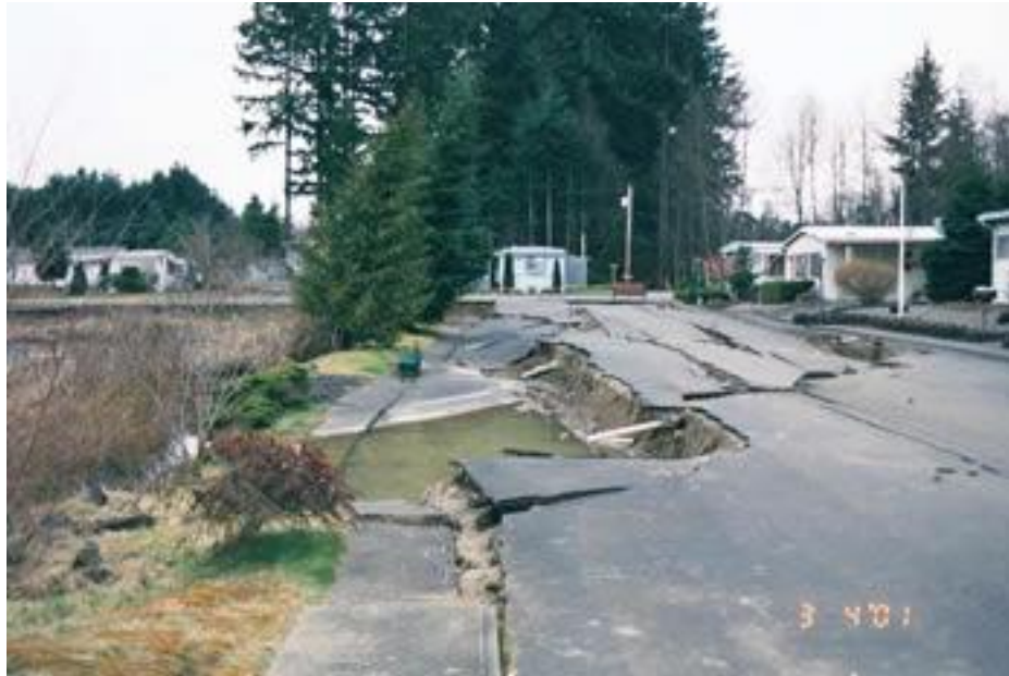
Figure 22. Liquefaction induced lateral spreading (courtesy of Geomatrix )
