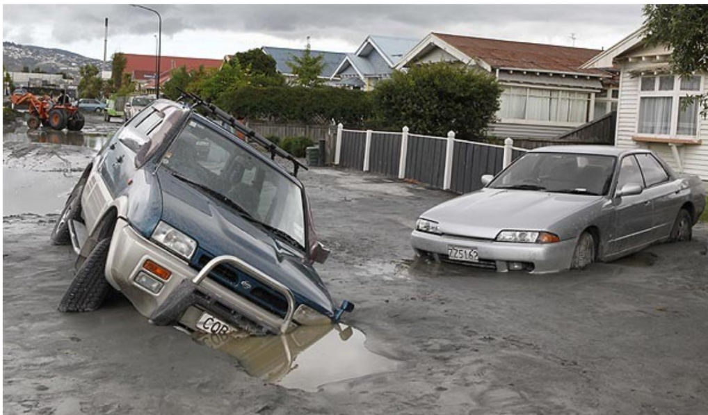
Figure 21. Effects of liquefaction in New Zealand, 2011 (courtesy of Temblor )
