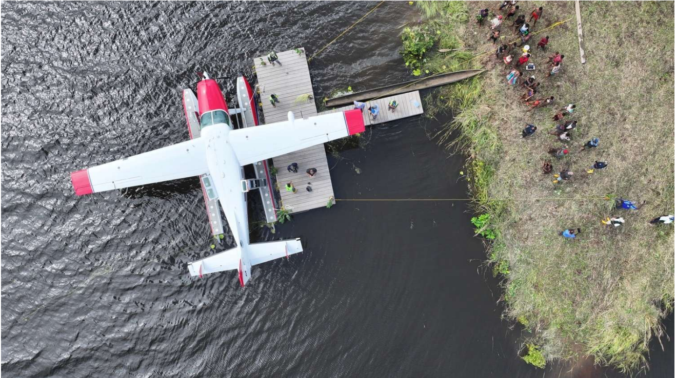
Fig 06. – Despite having recently experienced a 50-yr flood event, MAF is able to land their amphibious aircraft in Balimo, PNG with EMI-designed docking infrastructure that can adapt to changing climate conditions - maintaining a lifeline to this isolated community. (Photo by Terry Fahey)
