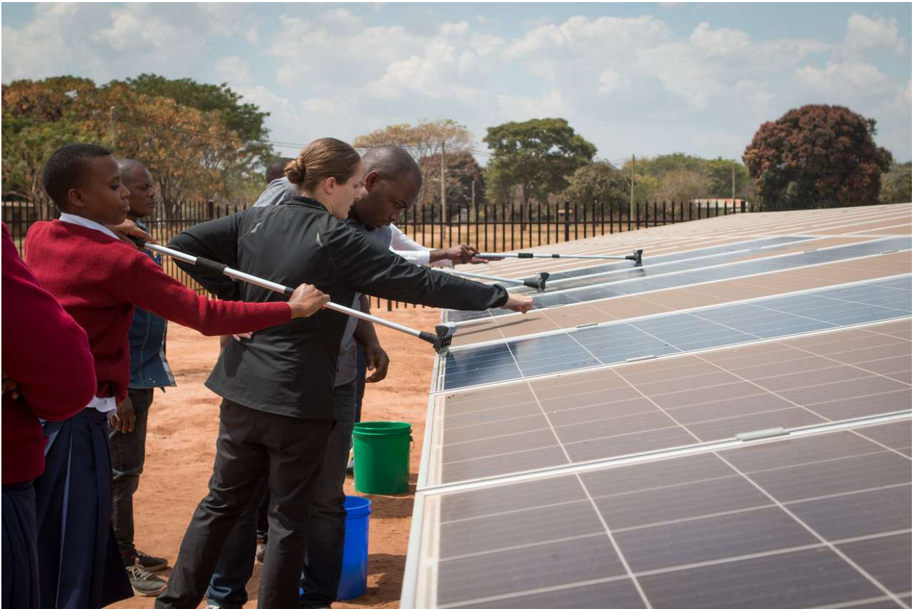
Fig 05. – Students learning how to clean and maintain solar panels from an EMI-designed micro-grid system for a campus in Tanzania (Photo by Jenni Keiter)
